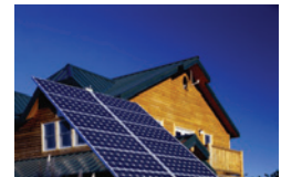
install solar panels
